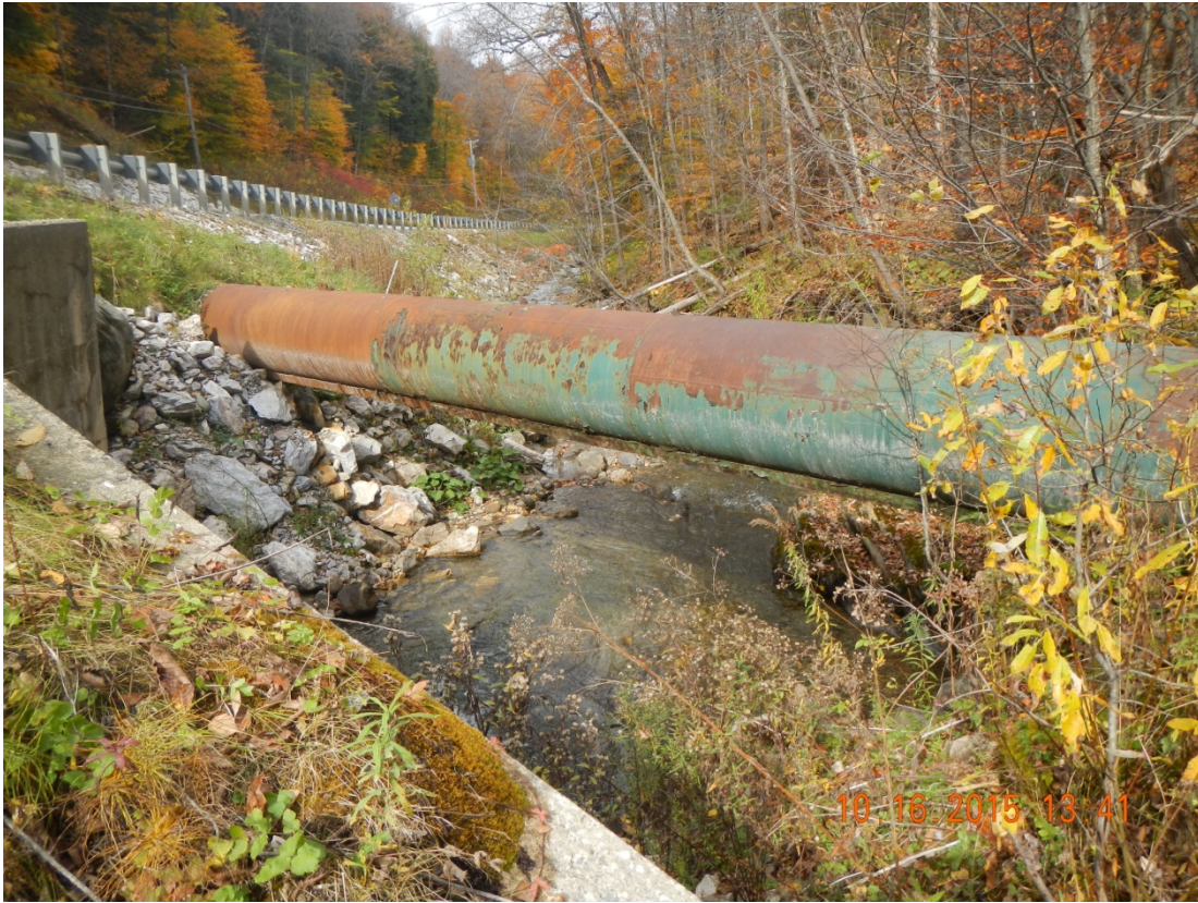
Figure 2: Water pipe Northeast of the Culvert Outlet
