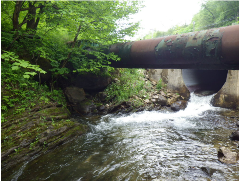
Picture 7: Outlet of Culvert, Exposed Bedrock in Streambed on Left
