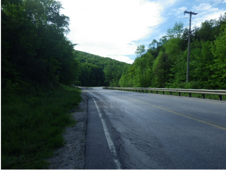
Picture 1: Bridge 115 – Looking South, Typical Top of Deck
