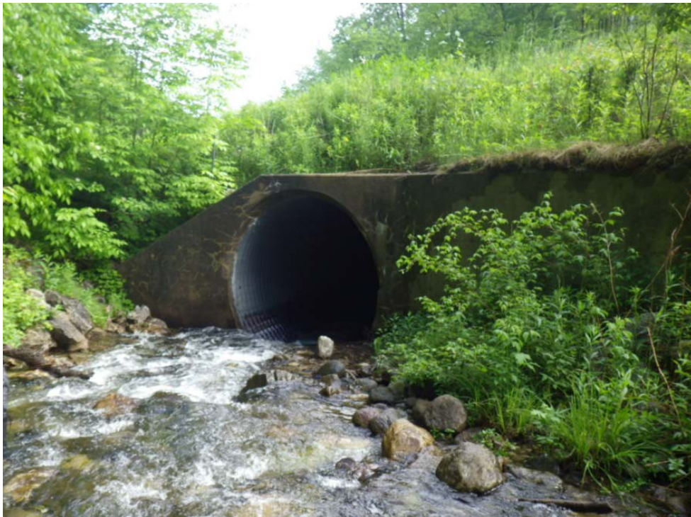
Picture 4: Inlet of Culvert, Stream Bed Steps Down into Culvert
