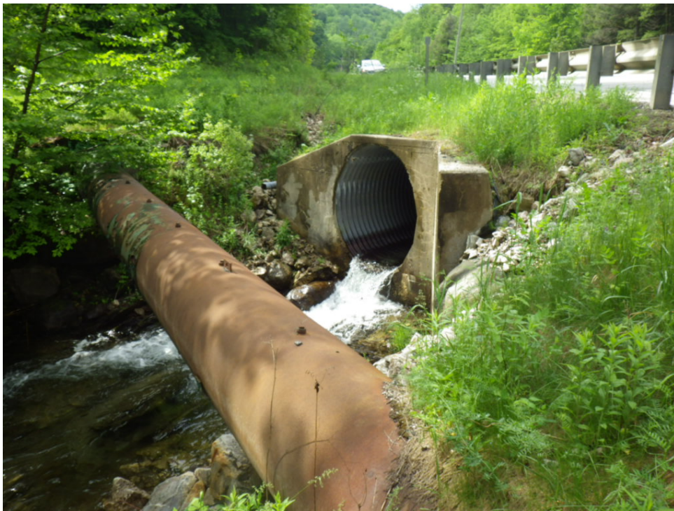
Picture 6: Outlet of Culvert, Water Pipe in Foreground
