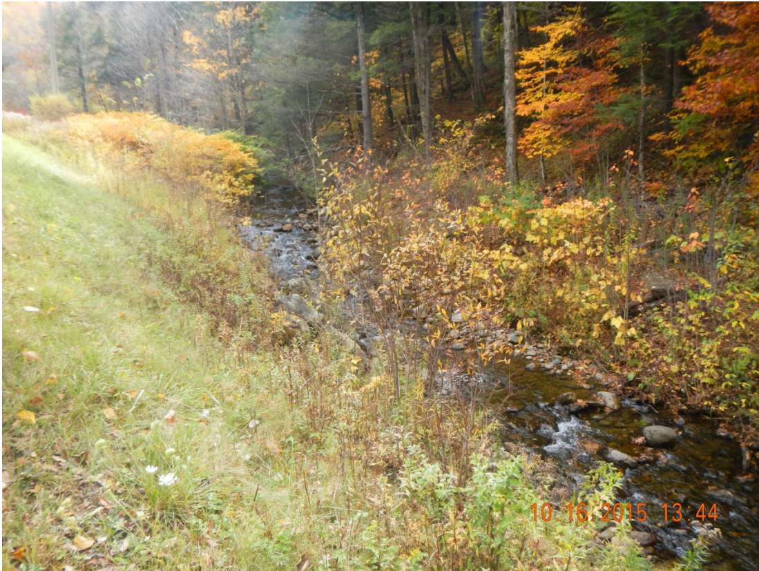
Figure 5: Boulders Upstream of the Culvert
