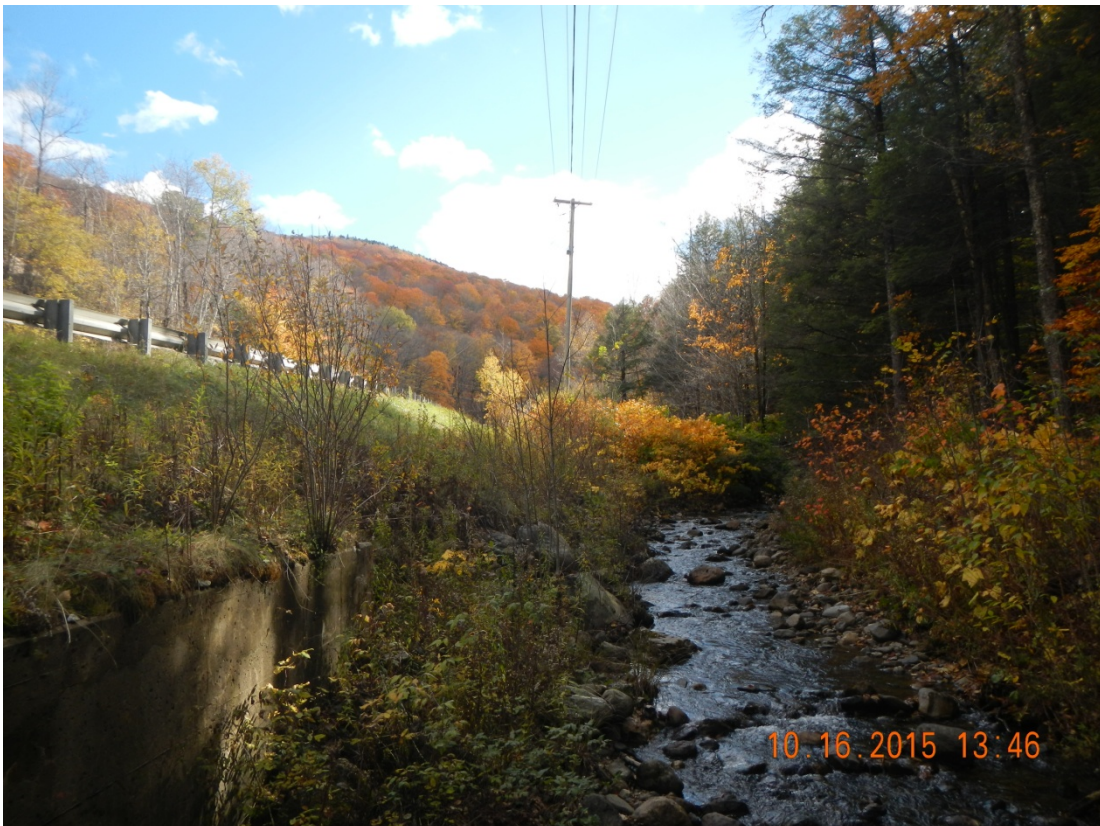
Figure 3: Utility Lines above Culvert Inlet
