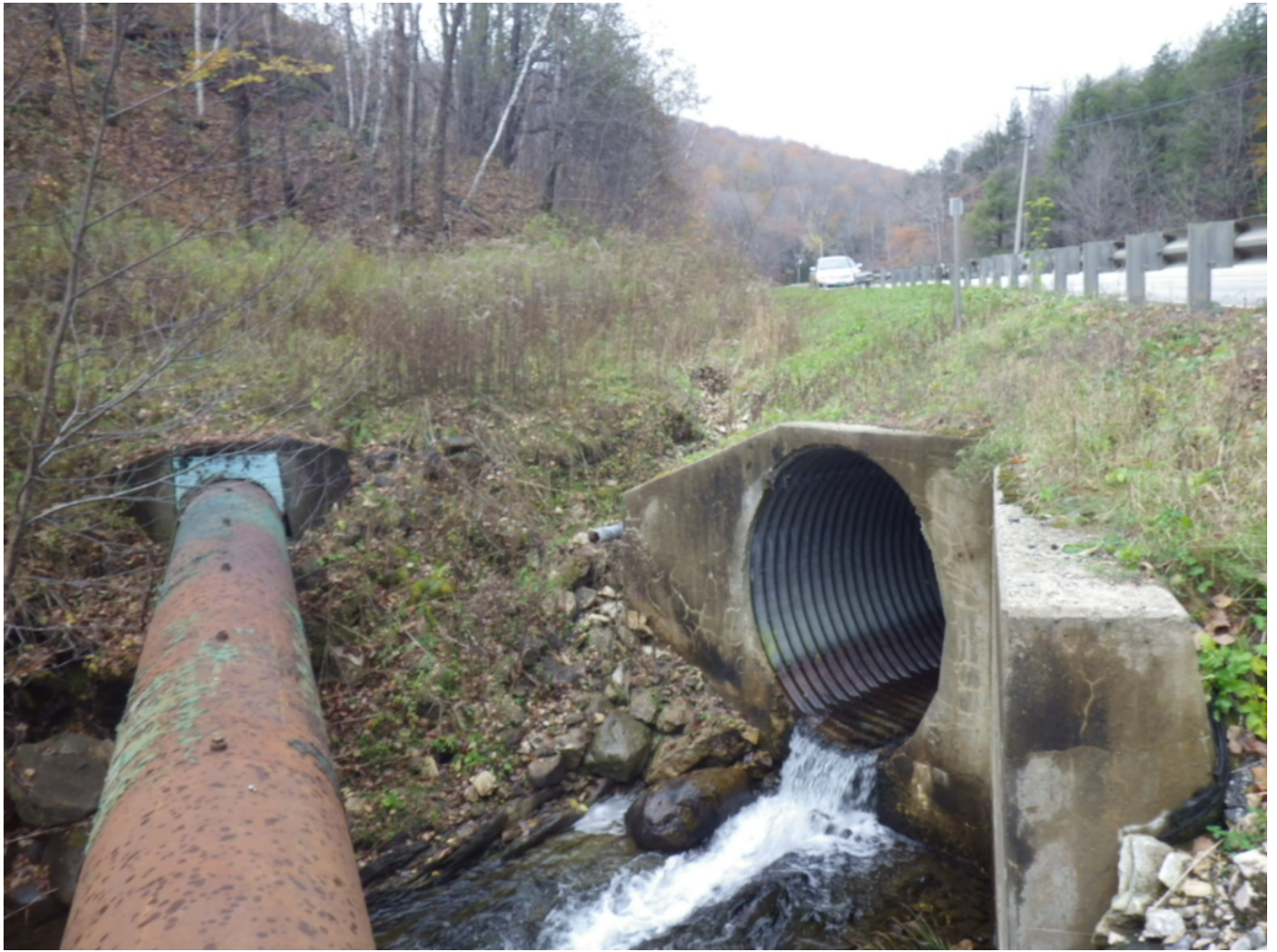
Figure 2. Bridge (Culvert) 115 at right with reinforced concrete head and wing-walls.
