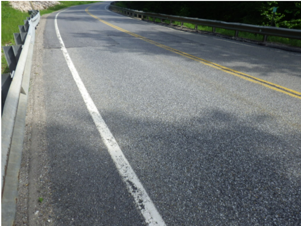
Picture 2: Bridge 115 – Looking North, Typical Deck
